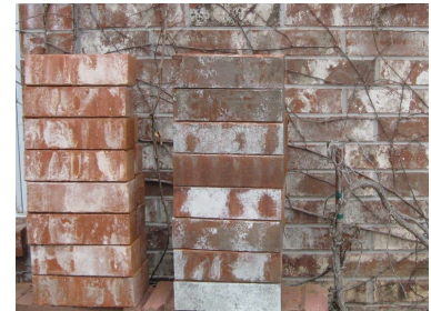
The stack of brick to the right used to look like the stack on the left. Wow!
